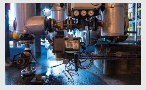
phragm actuator" applications, where corrosion or high vibration has required a better solution. One of the design features is a hollow shaft that enables passing long control valve shafts through and driving them from the top end, thereby providing a very compact valve and actuator package as compared to ½ turn diaphragm actuators.
