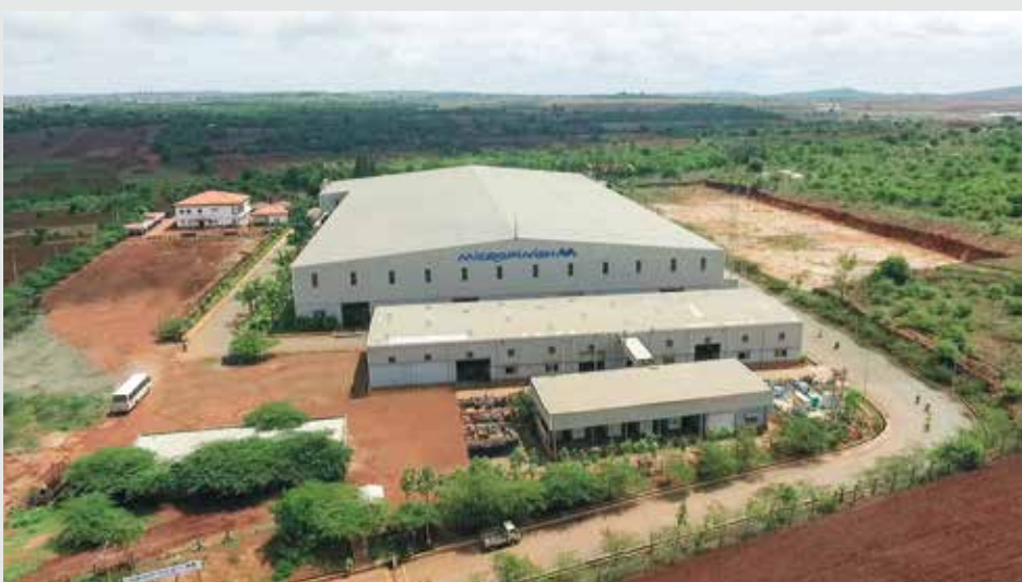
An aerial overview of the Itigatti facility.
